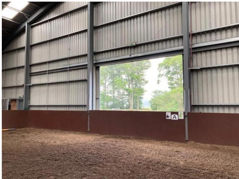
Picture One: A typical ventilation door (this building has seven) ensuring excellent natural ventilation
