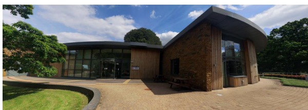
1 - View of the outside of the BHS HQ. There is brick paving up to the circular automatic doors. The outside is clad in wood and there are multiple glazed windows which are floor to ceiling.
