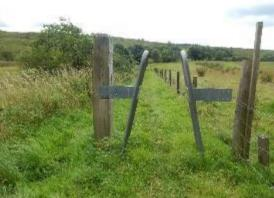
2 no. wooden footbridges over ditches/burns in line of path, bearers insufficient to support weight of horse
