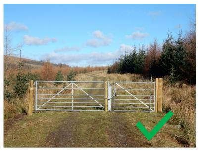
A side-gate minimum 1.5m wide adjacent to a locked gate, cattle grid or barrier will stop vehicles but still allow walkers, cyclists and horse riders access. Offset self-closing hinges will ensure the gate is stockproof. Commercially produced 1.5 m self-closing bridlegates with an integral H-frame are worth the investment to minimise future maintenance (available from
