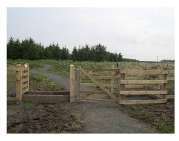
Provision of an adjacent kissing gate maintains unrestricted access for walkers. A RADAR gate would maintain access for wheelchairs too.
