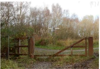
Elsewhere in Scotland, lockable vehicle barriers incorporating a horse stile have been used to good effect to restrict vehicular access whilst still maintaining equestrian access. The gap in the middle needs to be a minimum 1200 mm wide at the bottom and 2000 mm at the top. Timber rails over the lower section stop horses clanging their hooves on the metal.
