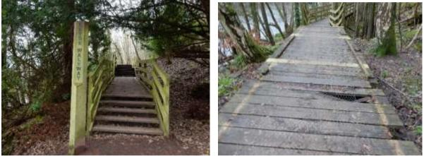
Between Mauldslie Bridge and Cardie's Bridge on the B701 there are numerous wooden footbridges, some only 90-100 cm wide, and some with rotten planks.
