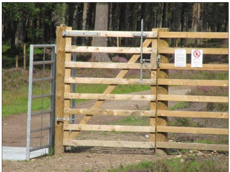
**Image 1 : Standard lever with high fixing point**
