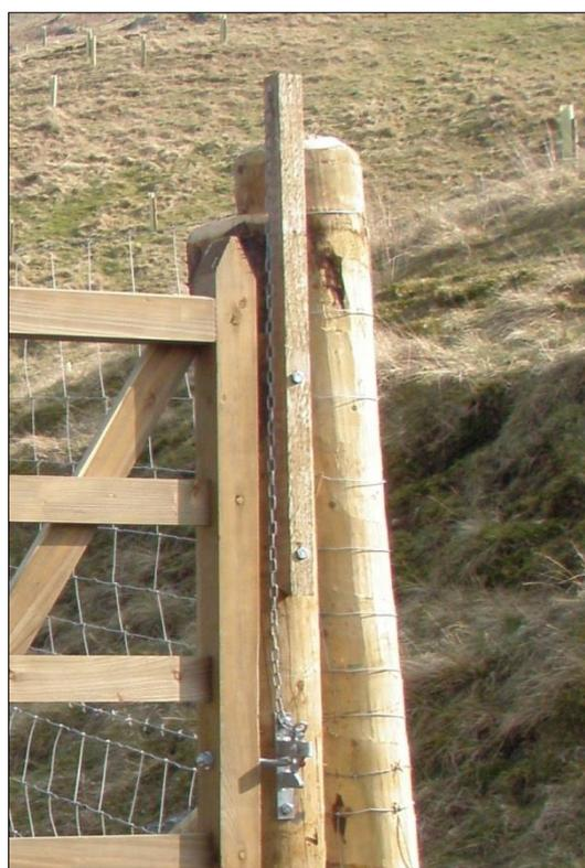
**Image 3: Chain extension to top of extra piece of wood. It would be better anchored to the top of the**
