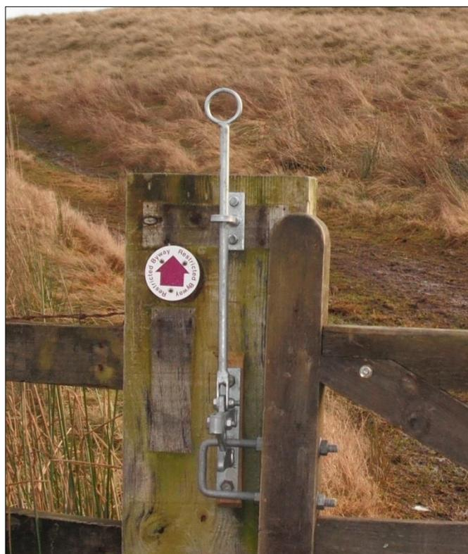
**Image 2: This ring pull is on an ordinary field gate but the same principle would apply to a deer gate.**
